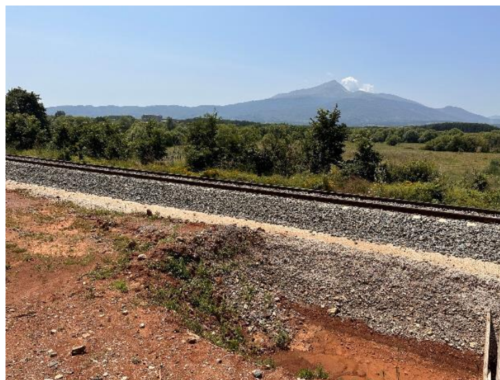
Figure 1-2: Photograph of planned WWTP location
